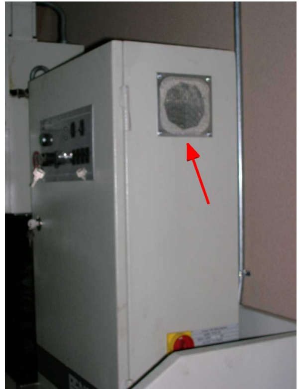
Upper vent screen mounted
