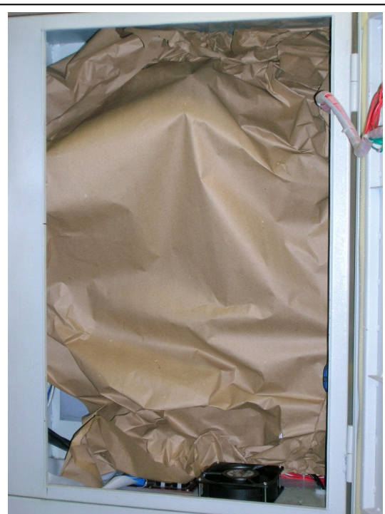
Shield the electronics from chips when cutting
