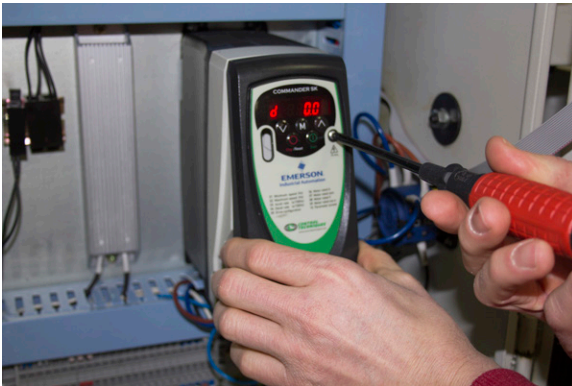
Figure 22: Removing the faceplate from the VFD.
