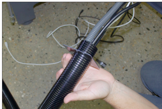
Figure 4-188: Loose end of corrugated tubing and all cords put through the access panel.
