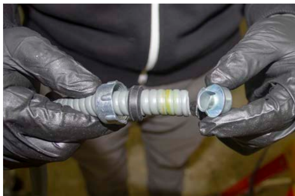
Figure 6: Flex conduit fitting assembly.
