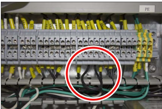
Figure 4-138: Example of the jumper wire on the terminal block.
