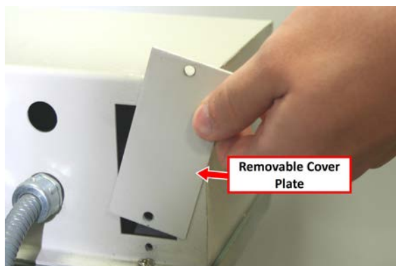
Figure 7: Cabinet-top box cover plate.
