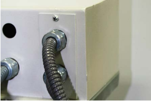
Figure 9: New cover plate installed onto the cabinet-top box.
