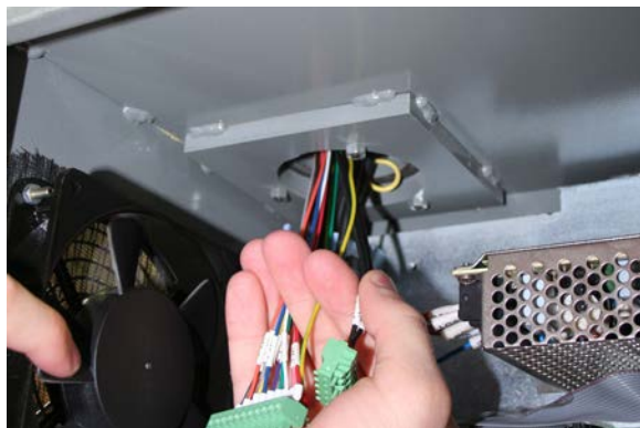
Figure 8: Power and encoder wires pulled into the electrical cabinet.
