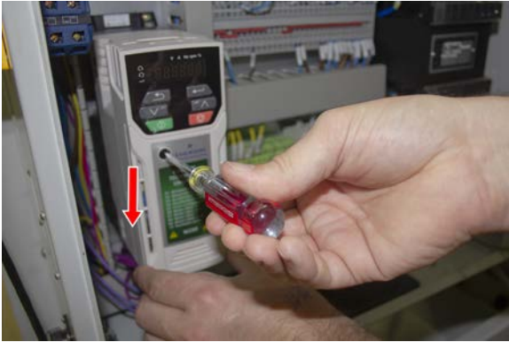
Figure 12: Removing the cover from the VFD.
