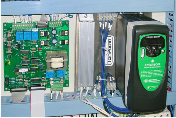
Figure 5: Replacement VFD installed.
