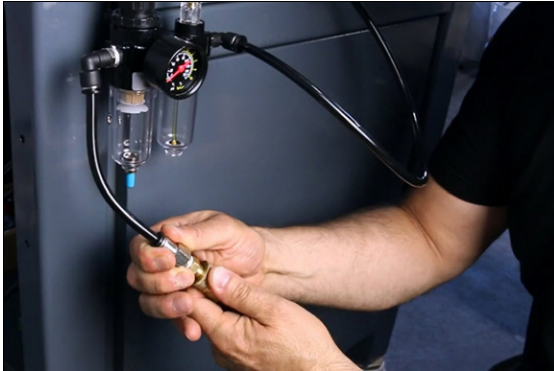
Figure 4-87: Connecting the air compressor's air line to the FRL.
