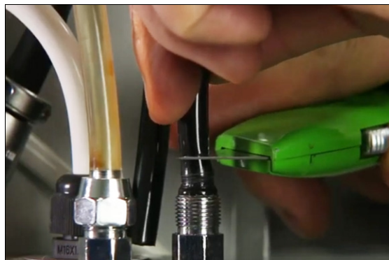
Figure 4-46: Cutting the water lines from the fitting.
