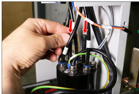
Figure 4-50: Shipping bolts installed on the top of the spindle.
