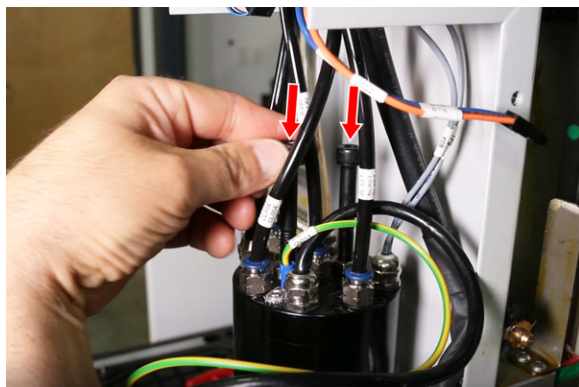
Figure 9: Shipping bolts installed on the top of the spindle.
