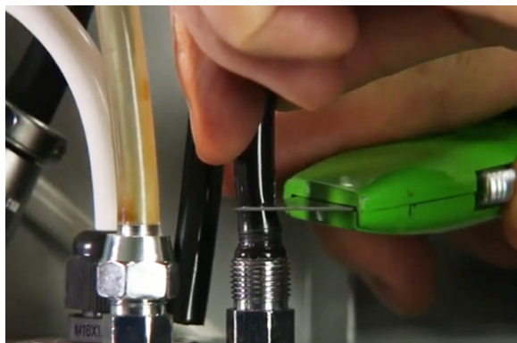
Figure 5: Cutting the water lines from the fitting.
