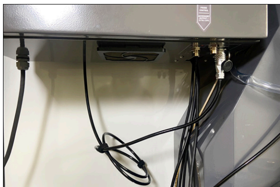
Figure 4-269: Cable connection made and secured with Velcro cable ties.
