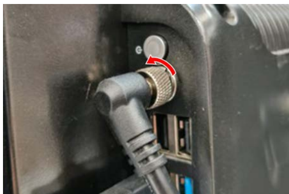
Figure 4: Removing the existing power supply cable from the console.
