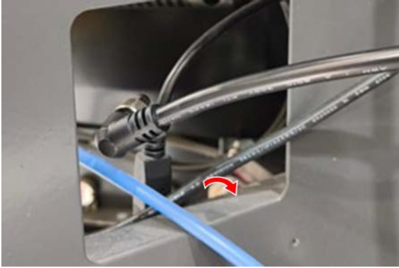
Figure 5: Removing the existing power supply from the rear access panel.
