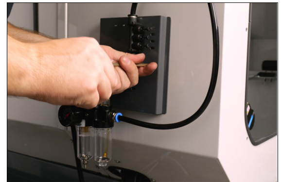
Figure 5-24: Installing the pressure regulator panel.
