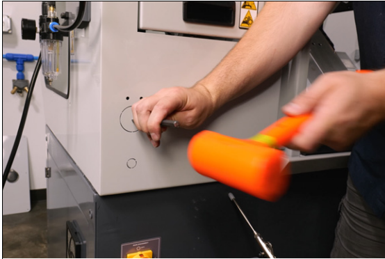
Figure 5-20: Removing the knockout panels on the front of the enclosure.
