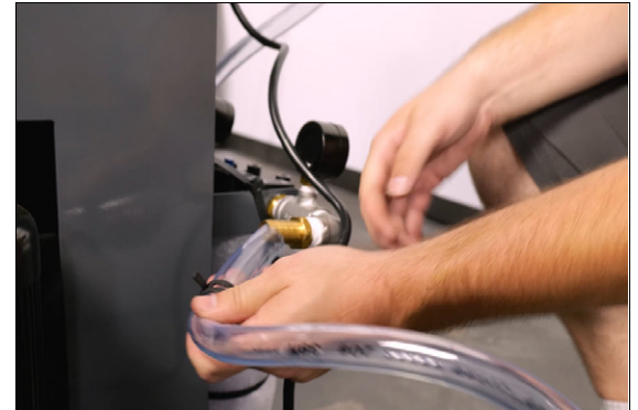
Figure 5-15: Connecting the coolant hose to the coolant filter.
