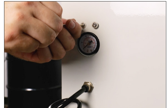
Figure 5-23: Installing the pressure regulator.
