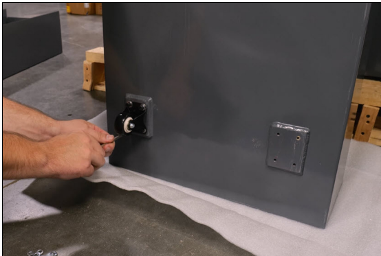
Figure 5-13: Installing casters on the coolant tank.
