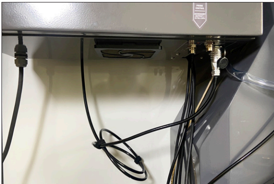
Figure 4-118: Cable connection made and secured with Velcro cable ties.
