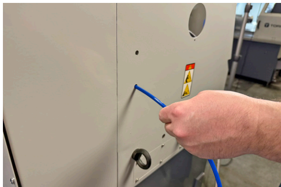
Figure 13: Routing Hose 3 through the access hole in the enclosure.
